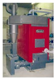
Figure 1-11: Boiler of 130-250 kW capacity (Binder, sold in Austria)
